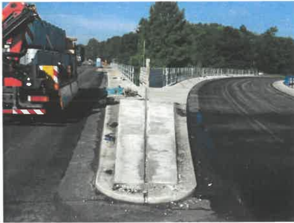
Installation of anchor plates / front
