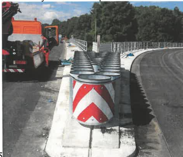
5 Crash cushion of the VECU STOP system on BW top cover
