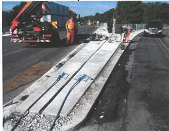
Installation of anchor plates / front
